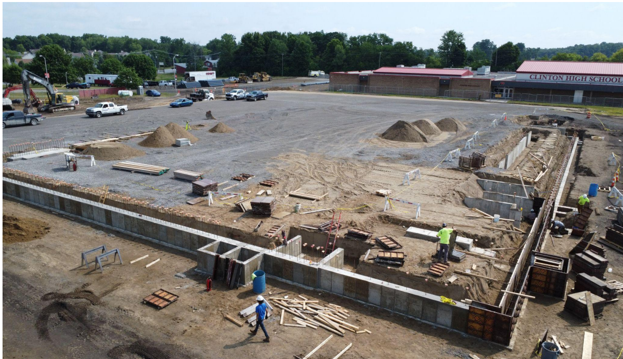
View from the West masonry contractor, with the gym wall block starting.
