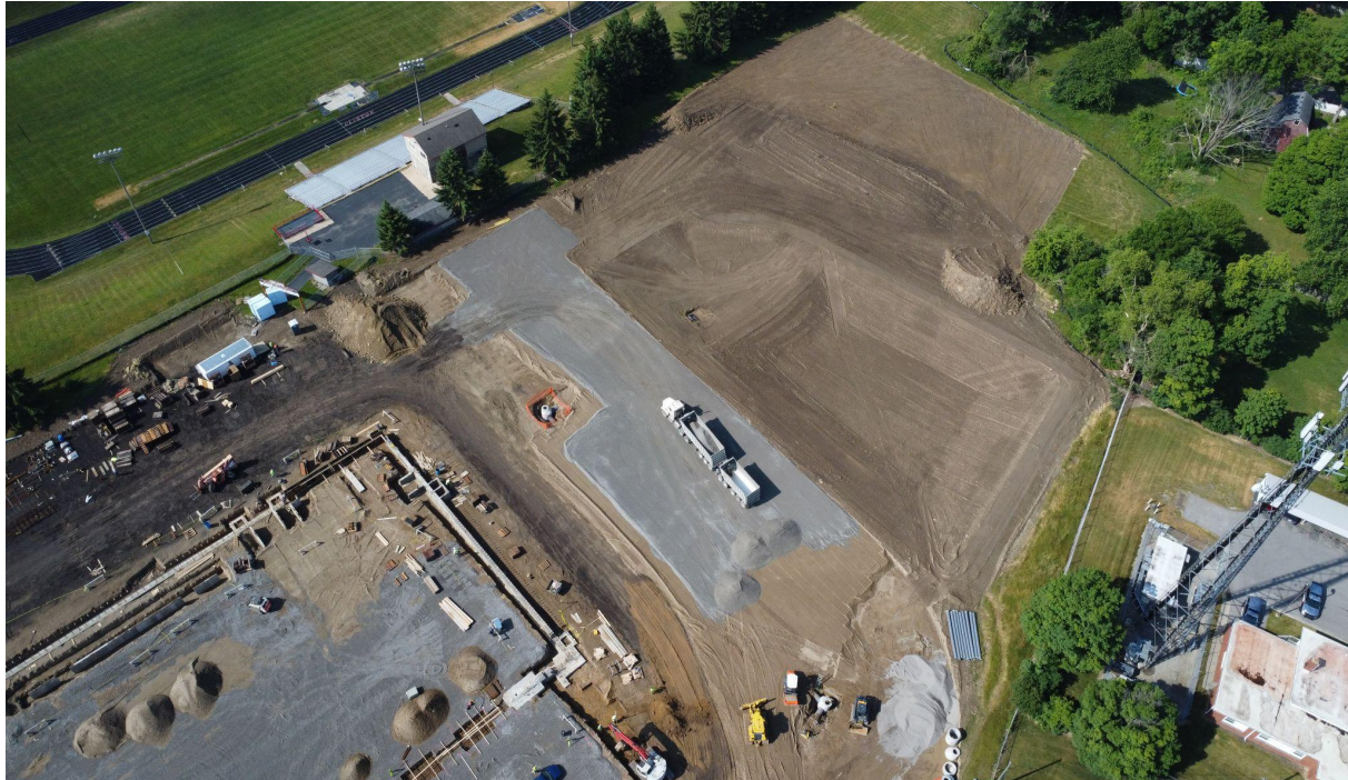
Aerial of the retention pond
