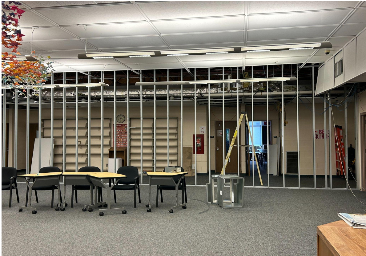
Wall/Hallway being added separating 2 buildings
